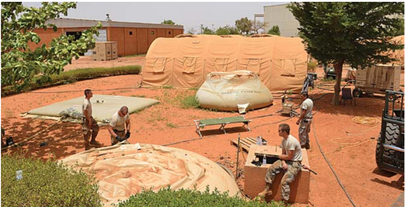
Det 2 Civil Engineers Senior Airman Thomas Bailey, Senior Airman Matthew Wallis, Airman 1st Class Ryan Ishmael, Tech. Sgt. Anthony Zhuckkasee (left to right) prepare to modify the existing water system to increase storage availability. (U.S. Air Force photo/Capt. Jeff Fowlkes)
