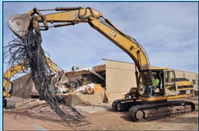
Creating sustainable installations is aided by the removal of outdated, inefficient facilities such as this building at Schriever AFB, Colo., that was demolished in late 2012. (U.S. Air Force Photo/Dennis Rogers)
